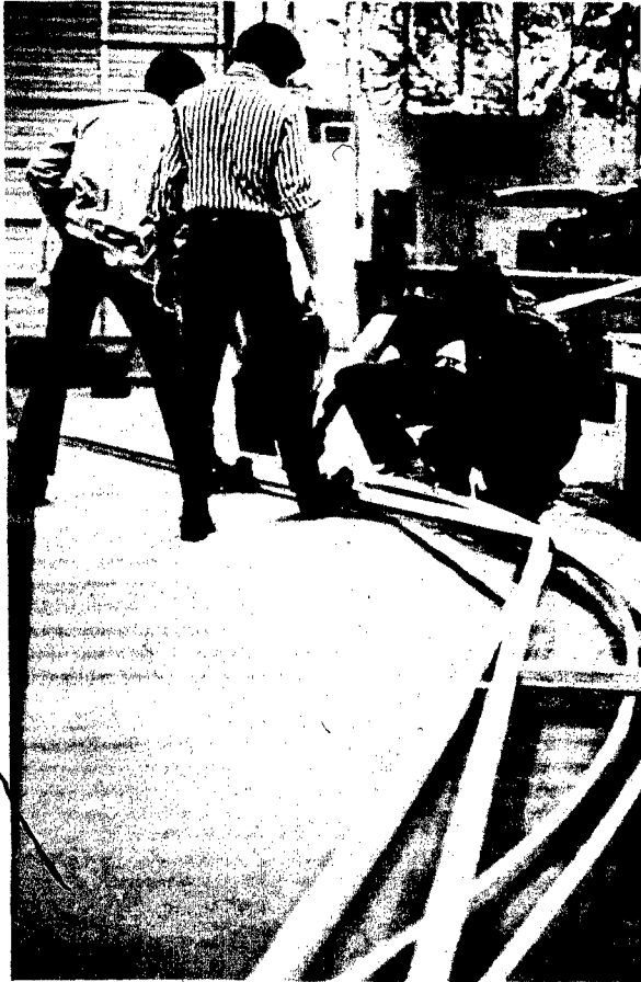
CARHART'S LUMBER was the scene on Thursday, March 25, of a construction project to build an arched dome in one night - and it was done! The dome, built by EAC members here with the help of Carhart's Dick Hammer, will be the Fair centerpiece.
